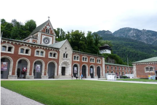
Alte Saline (Bad Reichenhall)
